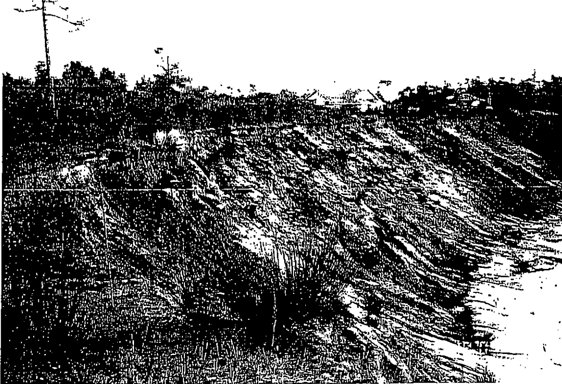
Location: Shelter Cove Subdivision - Siuslaw River Estuary, Florence, Oregon. Looking south from top of erosion bank. Note continuing massive slope failure. Also note distance to homes.
